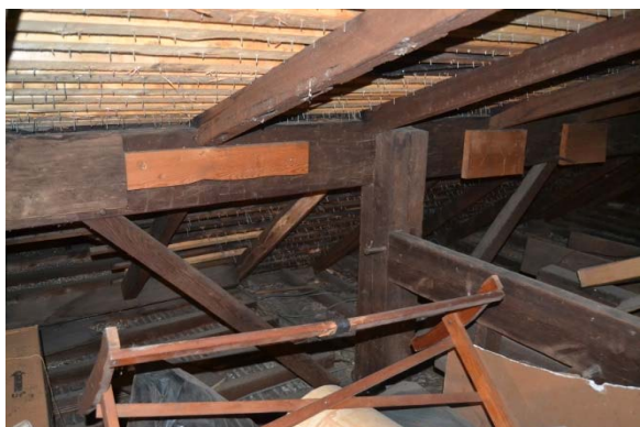
Photo 108: View in the attic of the north post in line with the wall on the east side of the hall.
