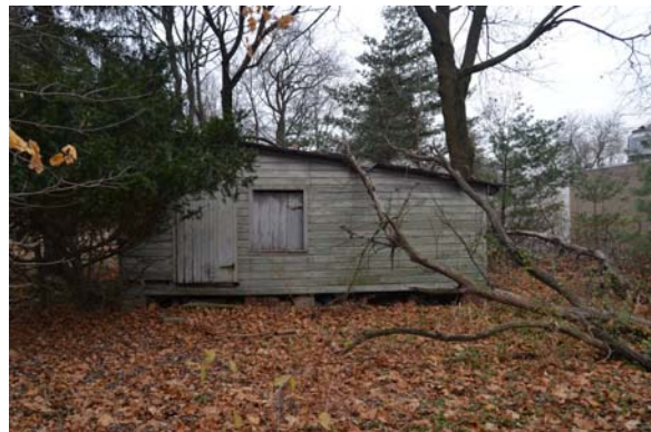
Photo 30: View of east elevation.
