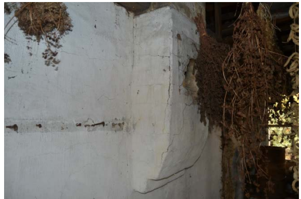
Photo 34: Close-up of the corbelled chimney base. Note thimble for a stove pipe.
