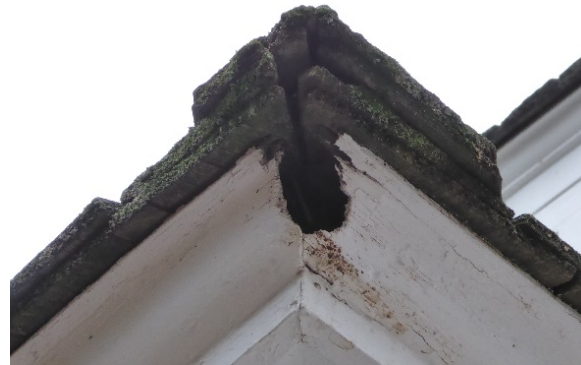
Photo 21: Hole in eave at right corner of porch roof.
