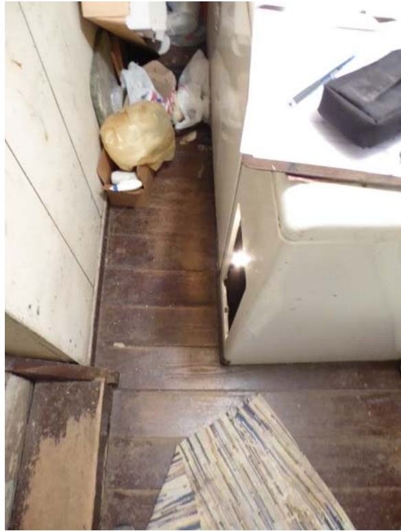
Photo 4: Flooring near bottom of stairs. Chest freezer at top right.
