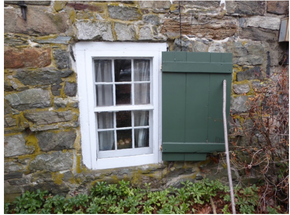
Photo 24: Basement window at main house. Bottom right piece of shutter missing. Biological growth at mortar joints. Iron tie rod visible at upper left.
