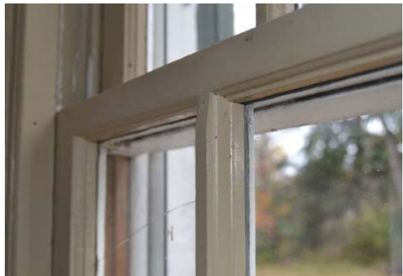
Photo 61: Close-up of one of the north window sash showing the replacement muntin, which is deeper than the sash and wider than the original muntin. Also note the small hole where a brad secures the muntin in place.
