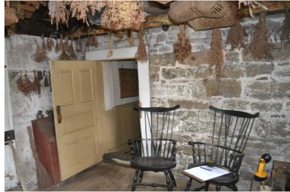
Photo 32: The west wall showing the door in to adjacent room. Also note worn whitewash on the stone wall.
