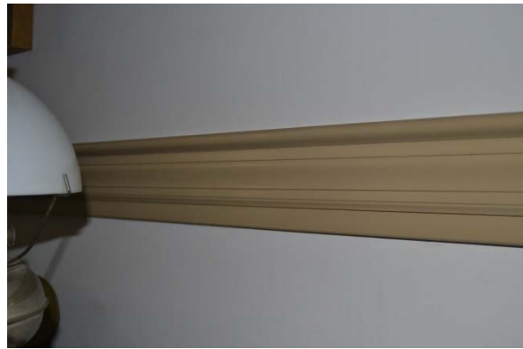
Photo 60: Close-up of the chair rail, which was added by the current owner.
