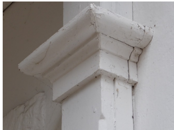
Photo 22: Right pilaster of porch has replacement piece at wall.
