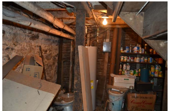
Photo 27: View into the east section of Room 001.
