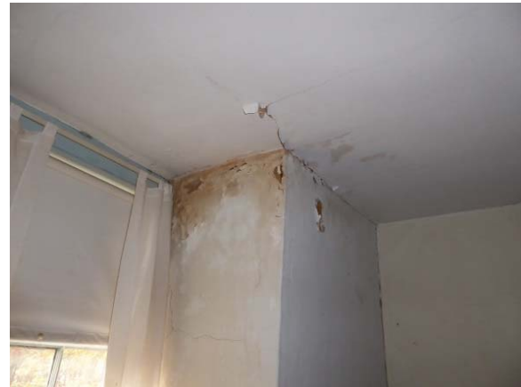
Photo 104: Plaster is failing at ceiling and walls of chimney bump-out.
