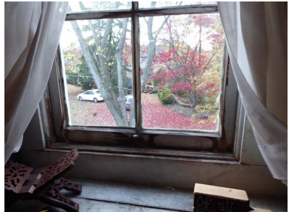
Photo 100: Detail of window. Wood has water damage.
