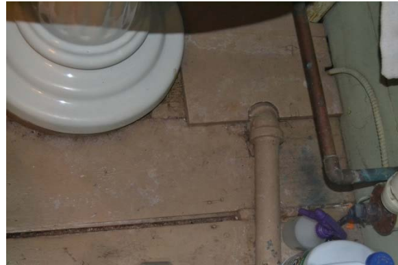
Photo 53: Condition of the floor next to the sink.
