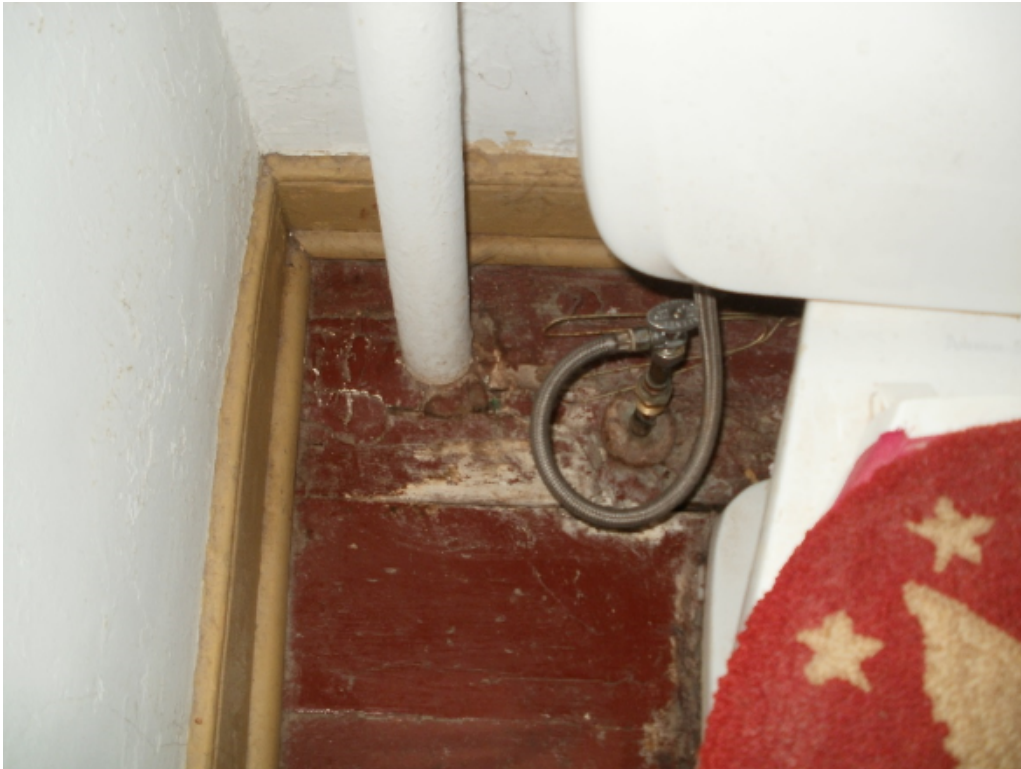
Water damage and failing floor in second floor bathroom
