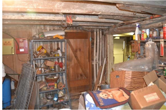
Photo 23: View southeast. Note wood ventilation slats on west wall and heavy joists ends from Room 002.
