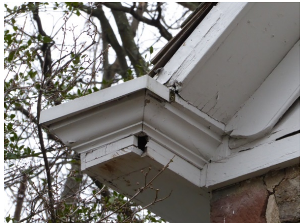
Photo 25: Left eave of gambrel roof at main house. Hole in corner of built-in gutter and rotted wood above cornice piece.
