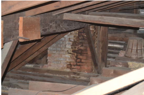
Photo 107: View of the northeast chimney. Note the water staining. It is not known if this leaking is active, but the flashing at the exterior and the roof appear sound.
