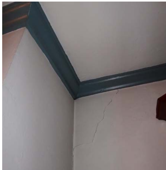
Photo 45: Crack in east wall to right of fireplace.
