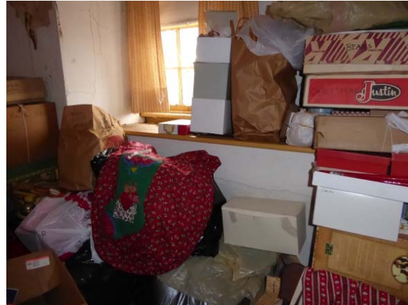
Photo 91: View west showing window and ledge. Crack runs length of wall below ledge.
