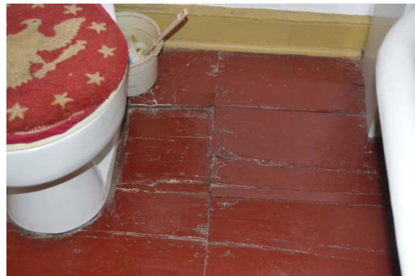
Photo 88: Area of damaged flooring around toilet in Room 206.
