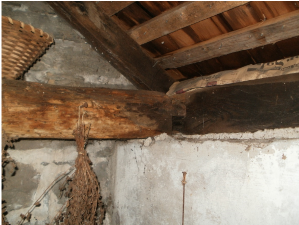
Separate mortise and tendon joint of smokehouse roof framing
