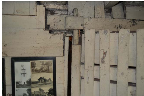
Photo 10: Close-up of the upper hinge at the slatted door. A block has been nailed over the female portion of the hinge to repair it. The rounded portion of the stile can slide up so the bottom can lift out to remove the door.
