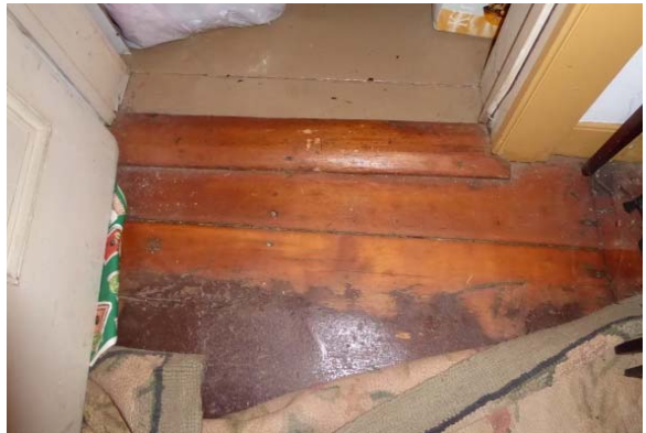
Photo 95: Wide board wood flooring with transparent and painted finishes.
