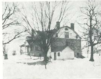
A New Jersey Colonial Farm House.
