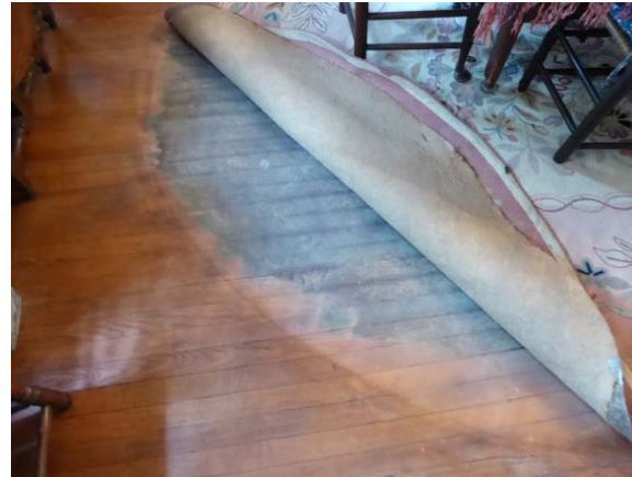
Photo 43: Narrow floorboards not original. Finish is worn and boards are stained under rug.
