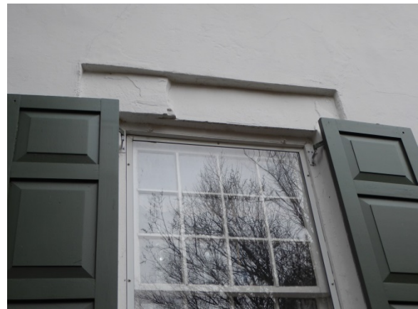
Photo 18: Piece has broken off stone lintel at left first floor window.
