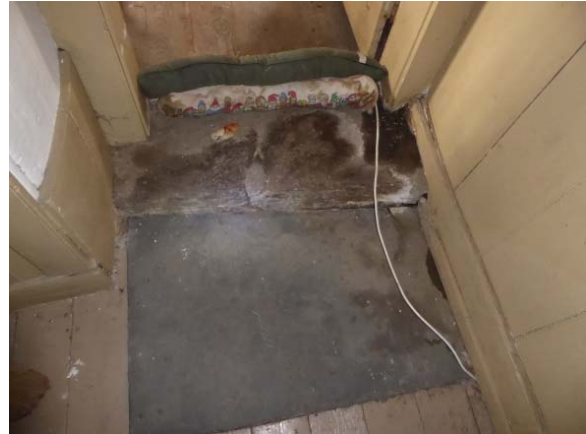
Photo 14: Stone slab and step up to smokehouse. Wood boards at side walls are bulging.
