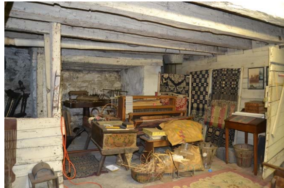
Photo 5: View looking northwest. The large fireplace foundation can be seen at the end of the room.
