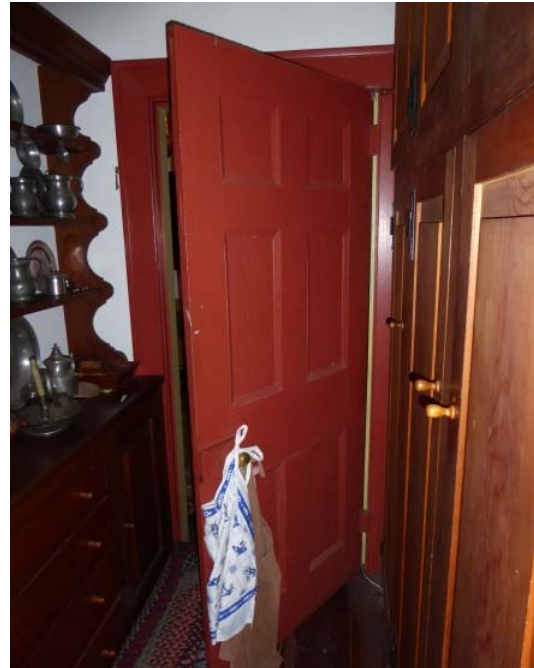
Photo 49: Door leading to hallway at west wall. Built-in shelves and cabinets to both sides.
