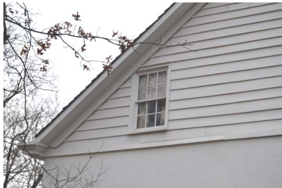
Photo 13: View of the north gambrel end roof slope and window.
