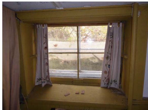
Photo 22: Window at north wall. Ledge is buckling and wood at right side is rotted.
