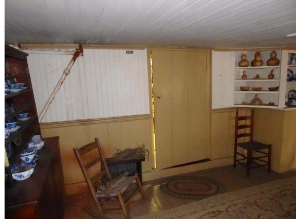
Photo 11: West wall with door to Open Cellar 002. Pipe at left is causing some water damage to wood.
