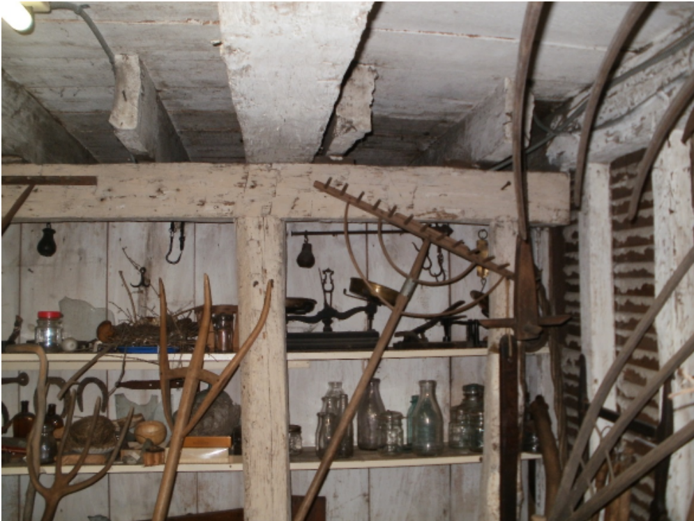
Varying floor joist depths and shims
