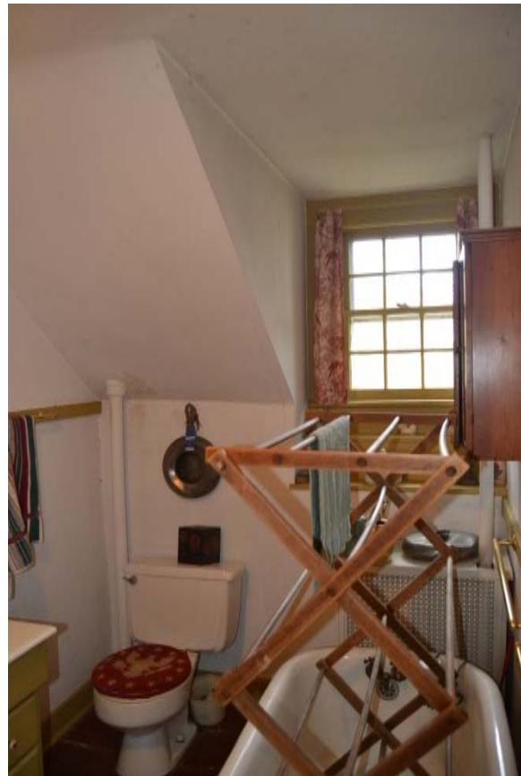
Photo 87: General view north. Note water damage at vent pipe next to toilet.
