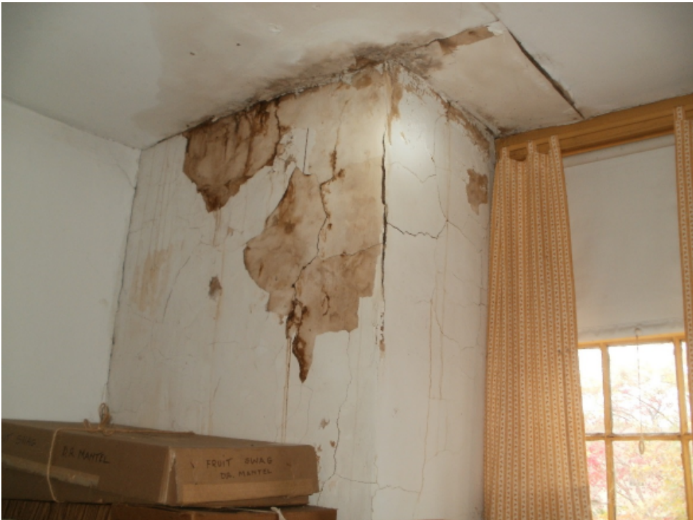
Water damage at west side north chimney
