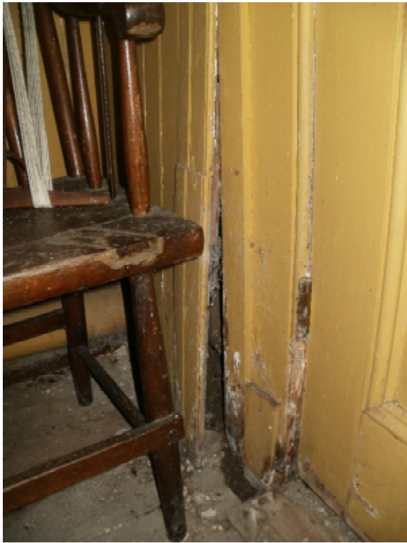
Northeast corner basement wall finishes displaced from water infiltration and wall debris
