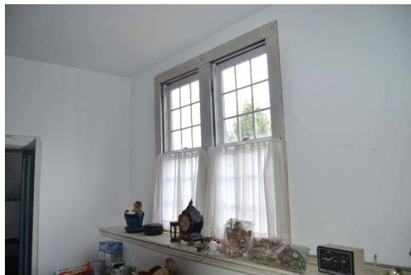
Photo 79: The paired window at the east gambrel end.
