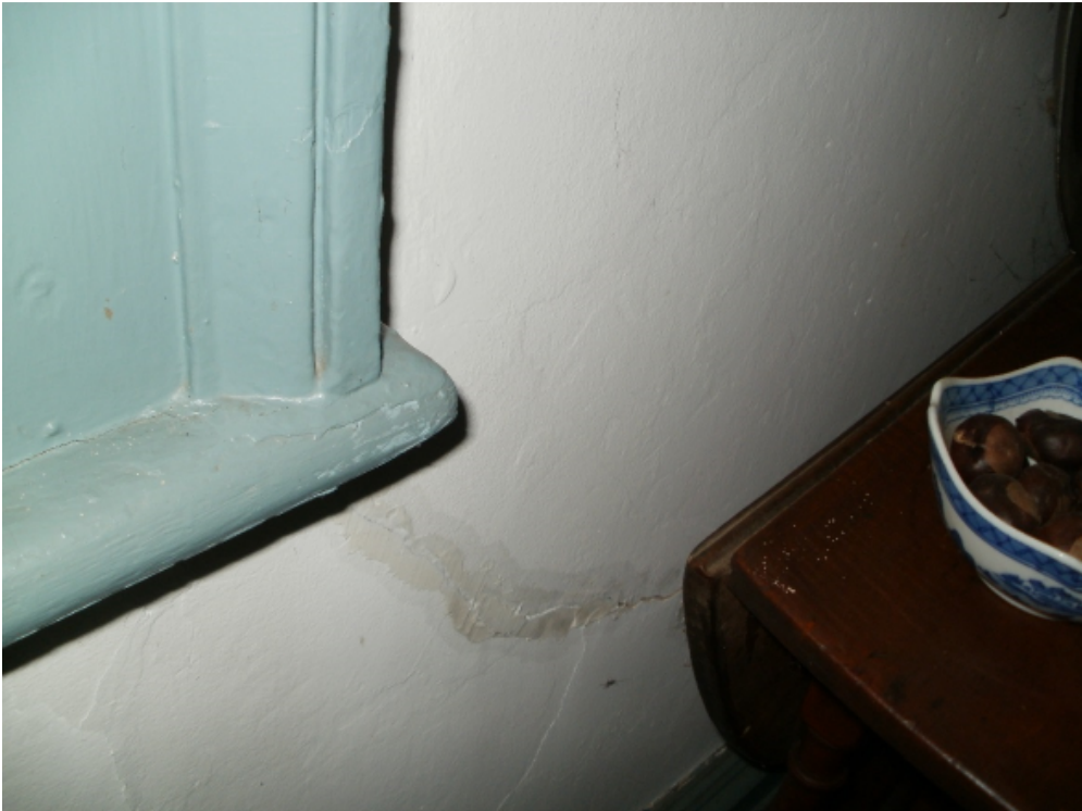
Typical cracks in plaster wall finishes
