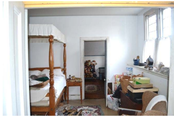
Photo 77: View north showing the door to Room 205. Note the shelf at right at the top of the exterior stone wall.
