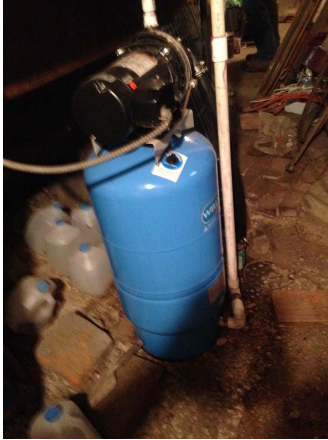
WELL PUMP AND TANK
