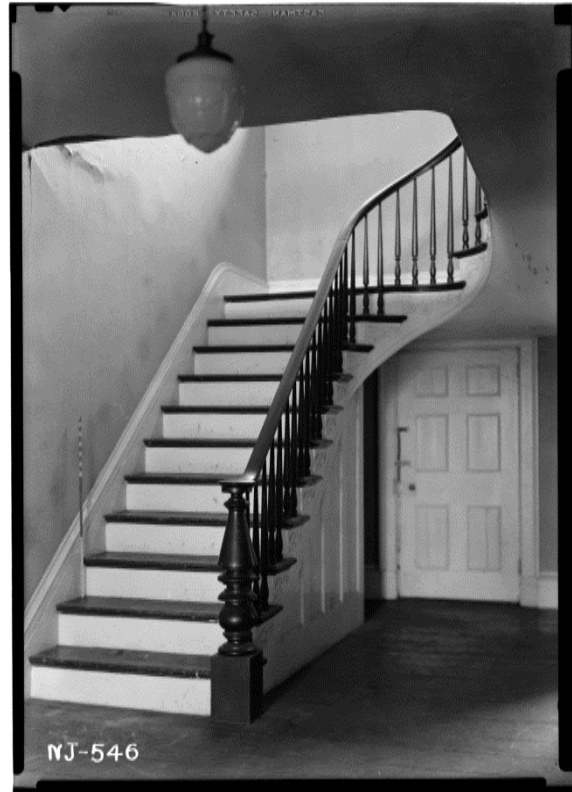
Photo 38: HABS photo of the stairs.
