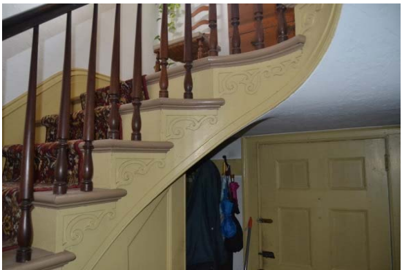
Photo 37: Scroll work at the face of the stringer at the stairs.
