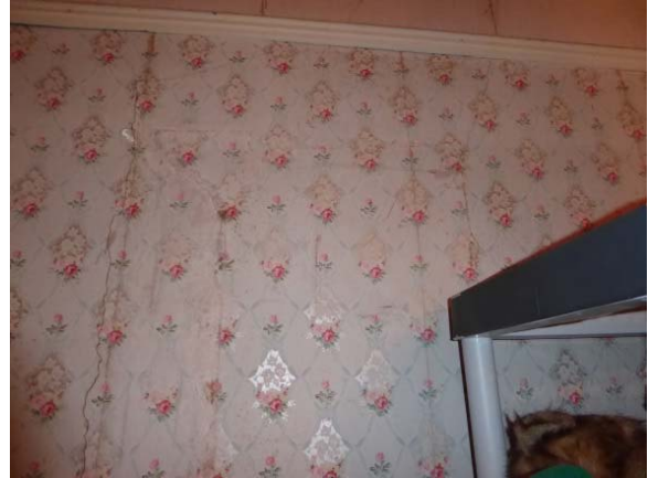
Photo 99: Cracks in south wall at left and square-shaped crack behind shelf indicating some kind of panel behind the wallpaper.
