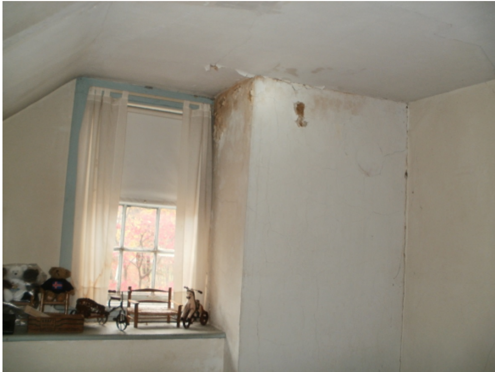
Water damage at west side south chimney
