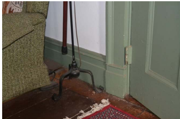
Photo 66: Detail view of baseboard and door casing.
