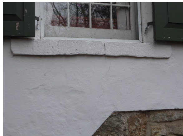
Photo 19: Crack in sill and wall at left window.
