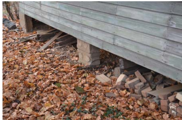
Photo 33: Detail of concrete block foundation piers..
