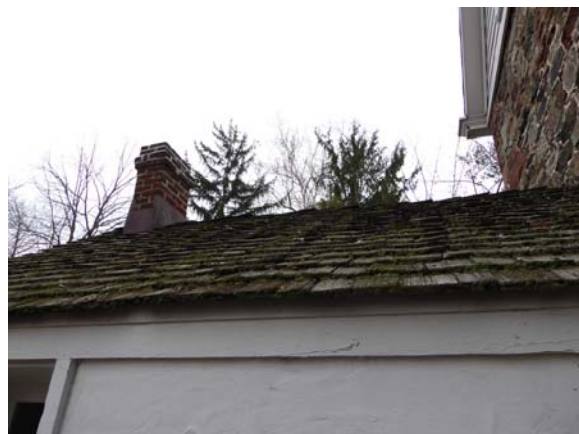
Photo 28: View of "smokehouse" roof. Shingles exhibit extensive biological growth and cupping.
