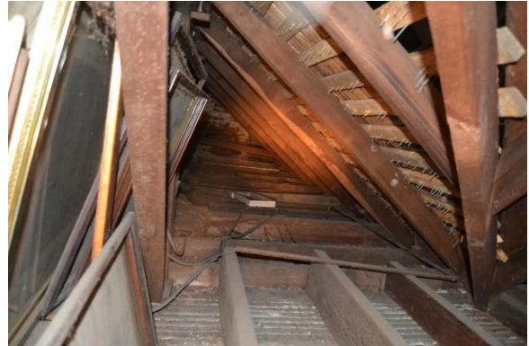
Photo 109: View east behind the line of the purlin. Note the roof pitch is steeper than in the above photos.
