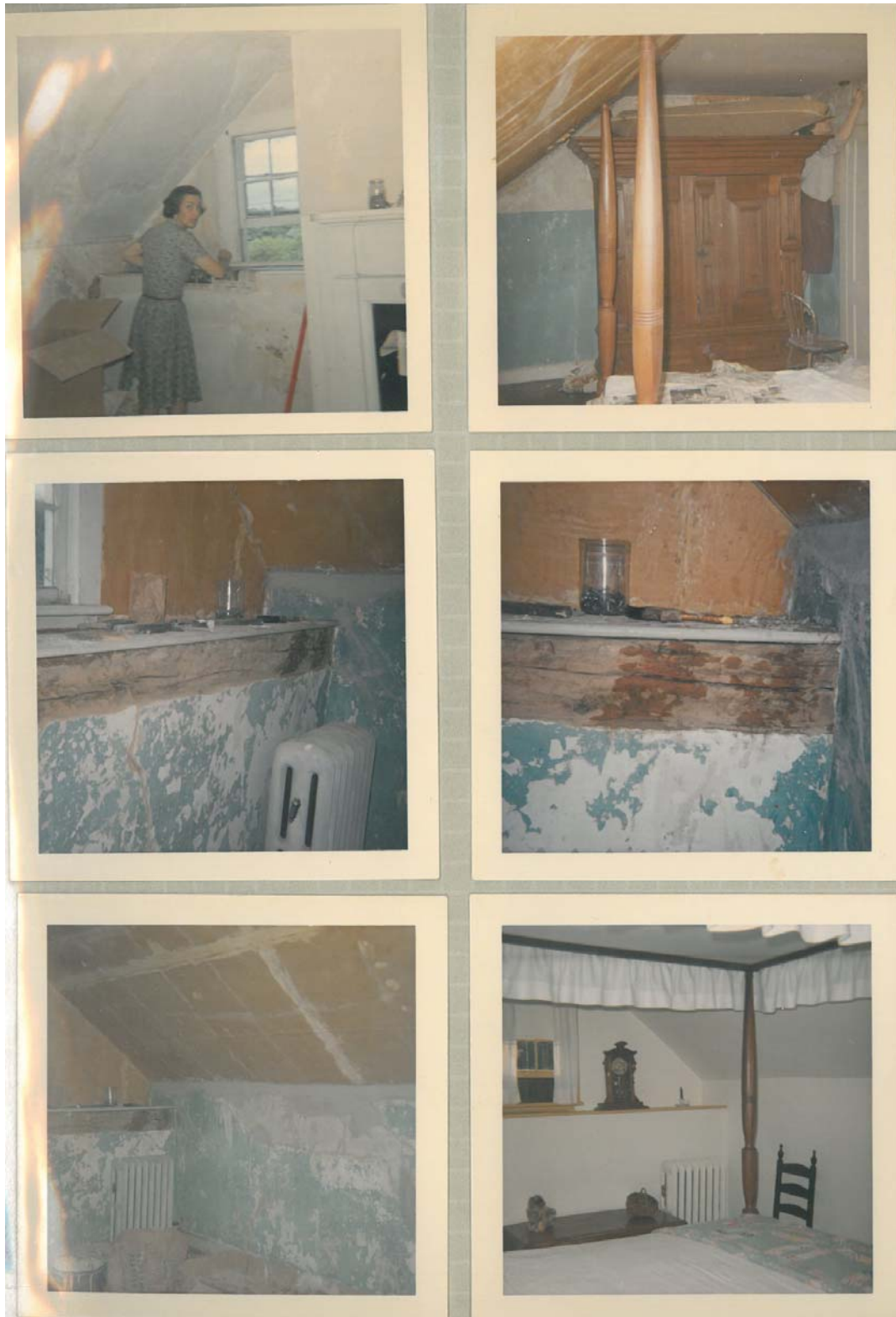
Figure 18: On the interior, they removed wallpaper, patched the plaster and repainted.
