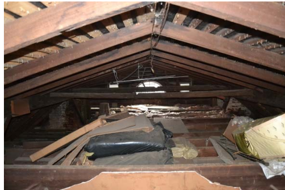
Photo 106: View towards east gambrel end. Water damage to wood is visible.
