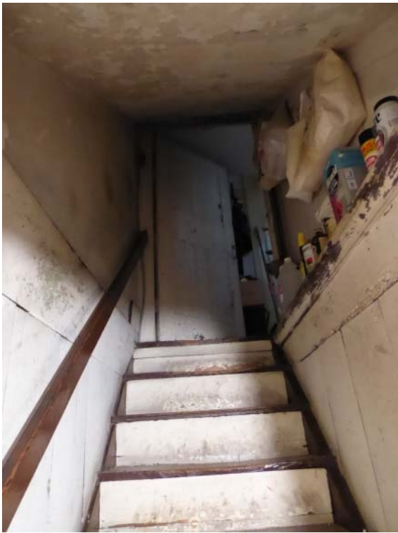
Photo 3: Looking north up basement stairs. Plaster ceiling peeling and stairs worn.
