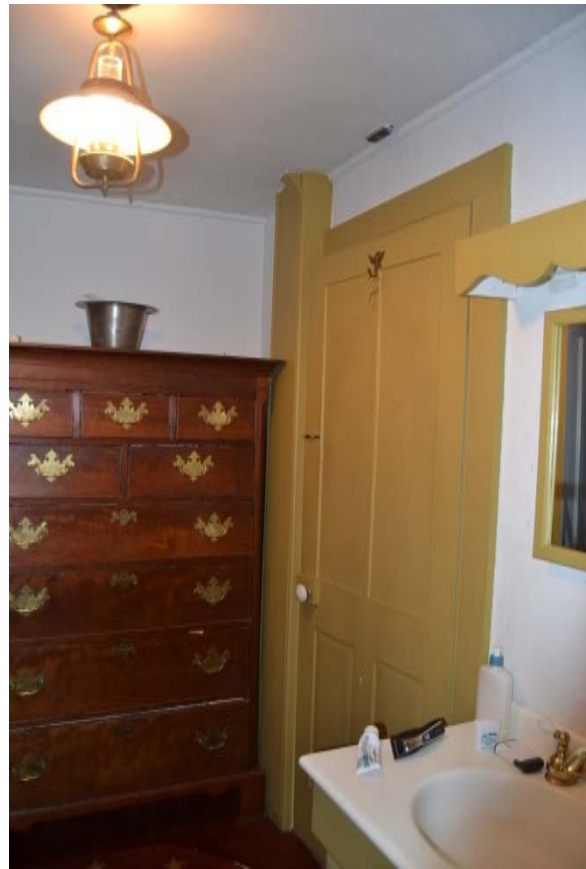
Photo 89: View south showing the door to the hall. Also note the cased out post immediately adjacent to the door.
