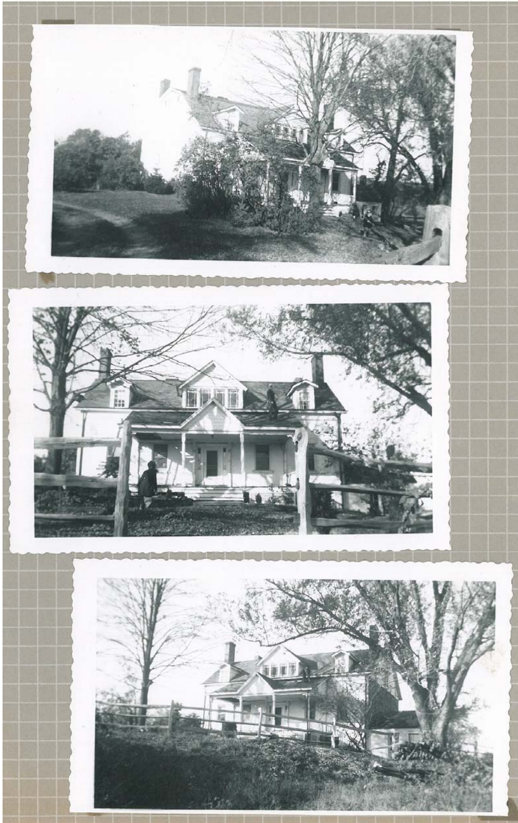
Figure 17: The Bogerts immediately set to work on the house. They replaced the roof and the porch.
