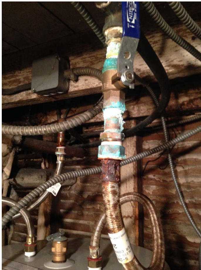
CORROSION AT WATER HEATER
