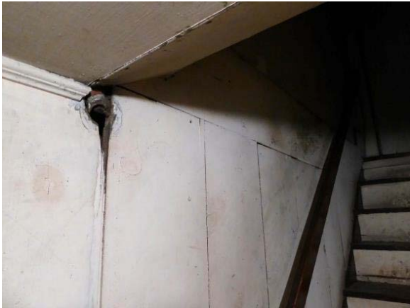
Photo 2: West wall of Room 001.
