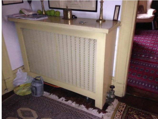
STEAM RADIATOR IN FOYER
