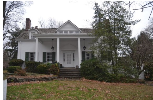
Photo 2: Direct view of the south façade highlighting the large Colonial Revival porch.
