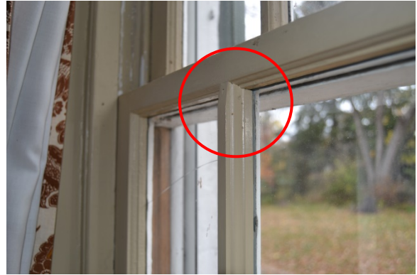
Photo 7: Detail of window interior. The thickness of the muntin, the taper where it meets the rail and the small nail hole all indicate that the muntin is a replacement.
