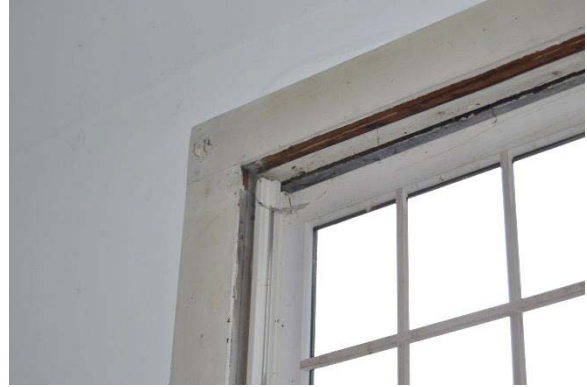
Photo 80: Close-up view of the window showing the replacement vinyl sash, the installation of which is poorly executed.
