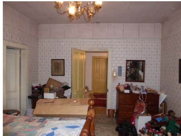
Photo 97: Door looking east toward stair hall.
