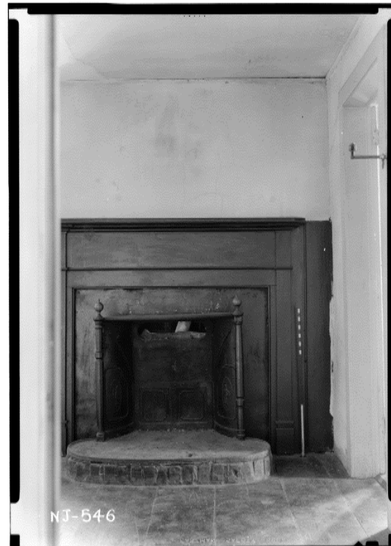
Photo 83: HABS photograph of the fireplace in Room 205. Note the addition of a raised hearth to accommodate the Franklin stove insert.
