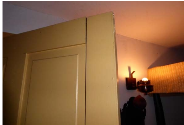
Photo 94: Door stile and rail are separating.
