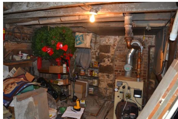
Photo 25: View west in Room 001.
