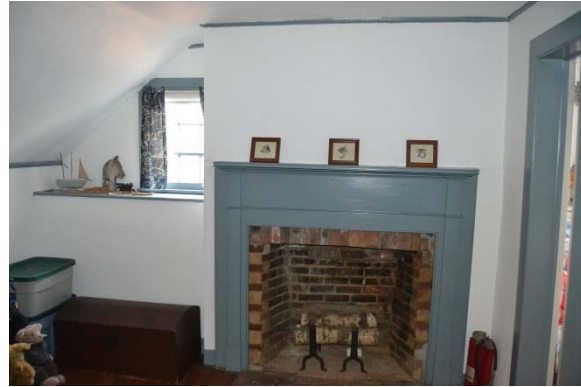
Photo 82: View east showing the fireplace and window at this end of the room. The small crown moulding is also present in the HABS photo.
