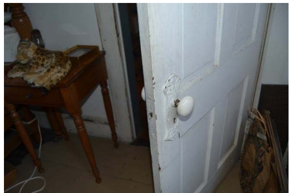
Photo 81: Detail of the door to Room 205. Note the door panel is different than is typical at the second floor. This door has a slight raised panel and a panel moulding that is integral to the stiles and rails.
