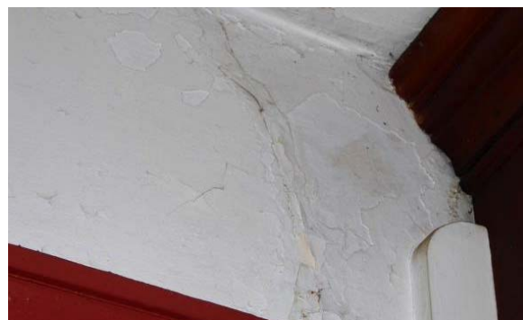
Photo 48: Crack in plaster above window at north wall.
