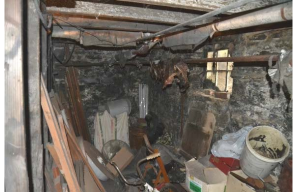
Photo 26: View into the northwest enclosure, which may have previously been a coal bin.
