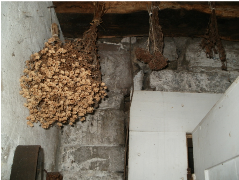
Missing mortar in stone wall above door from smokehouse
