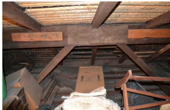
Photo 110: View of the joint of the two sections of purlin on the north side of the attic. The section of purlin to the right is hewn and that on the left is sawn, however this does not appear to be related to the roof being built in two sections.
