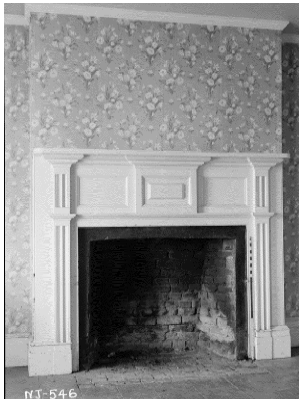
Photo 63: HABS view of the fireplace.
