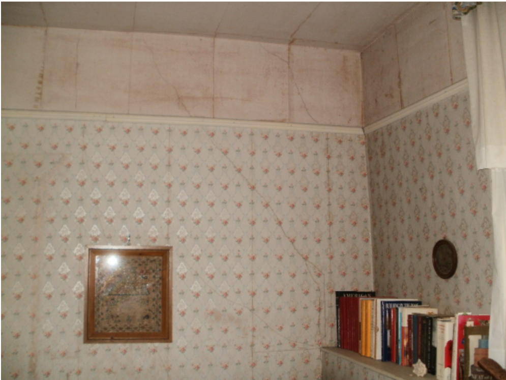
Typical cracks in plaster wall finishes
