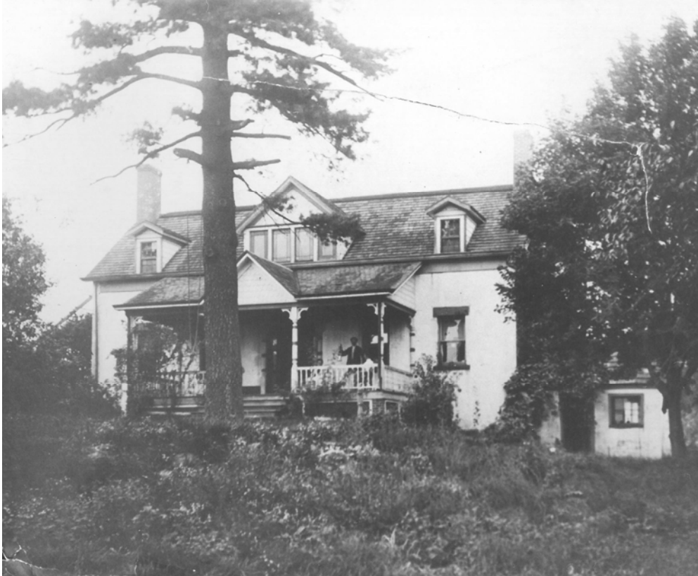
Figure 13: Undated photograph but presumed to be Lockwood May on the porch, therefore dating it to before 1896. Note the one-over-one sash, full porch, and large center dormer.
