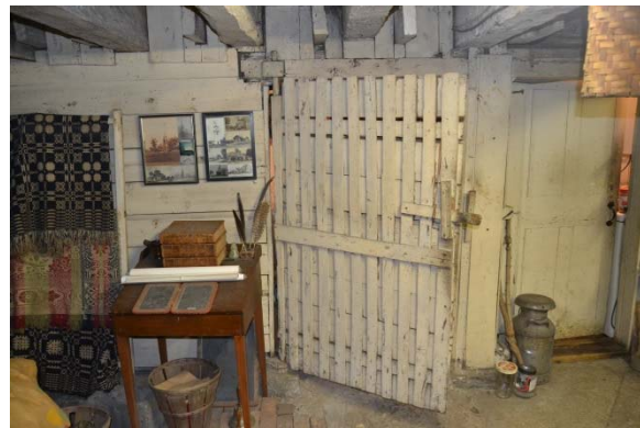
Photo 9: The slatted door to Room 001 is of very early construction.
