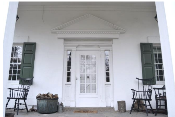
Photo 5: View of the front entry door. The pediment above the door represents later construction by the current owner, installed after the former porch was removed.
