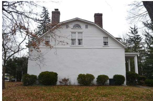
Photo 10: General view of the west elevation.
