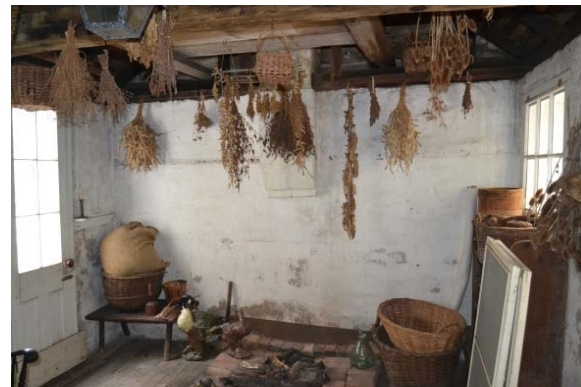
Photo 31: View east in Room 006. Note the chimney base corbelled out from the wall, rather than extending down to a foundation at the floor.
