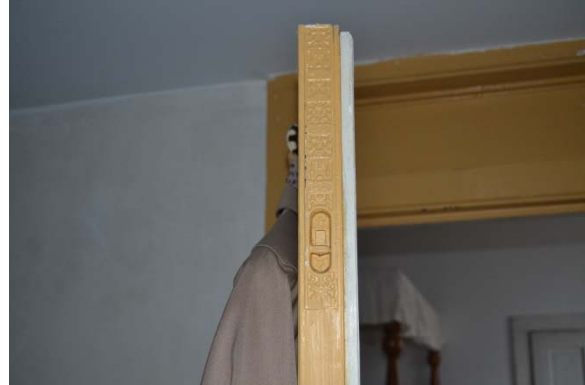
Photo 76: Detail view of the Victorian flush side bolt at the edge of the door into Room 204.
