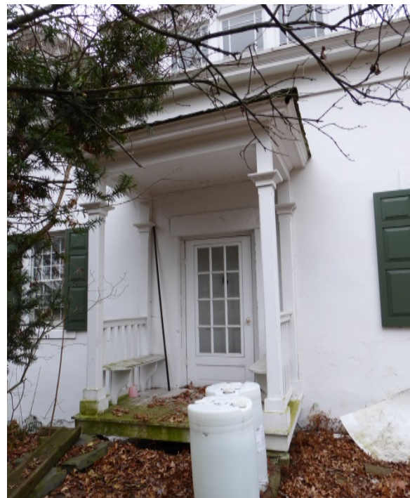
Photo 16: View of the rear entry porch and storm door. Biological growth on porch floorboards.
