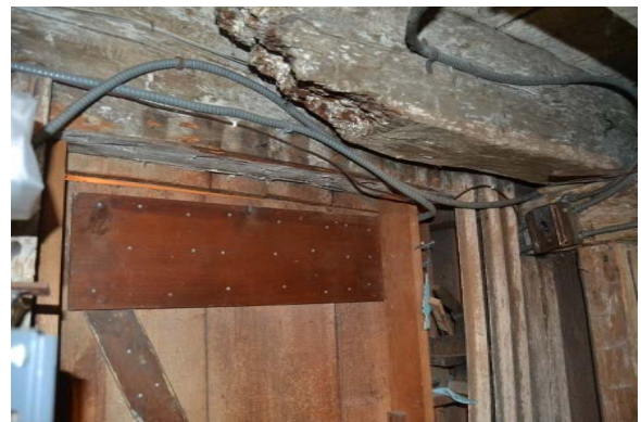
Photo 28: View in the southeast corner. Note the ghost marks of the slats above the door. Also note the deteriorated end of the large joist that extends into the room from Room 002.
