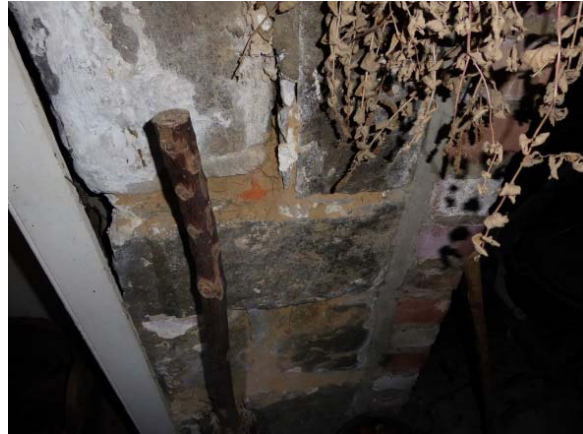
Photo 16: Stone to left of fireplace has powdered remains of plaster.
