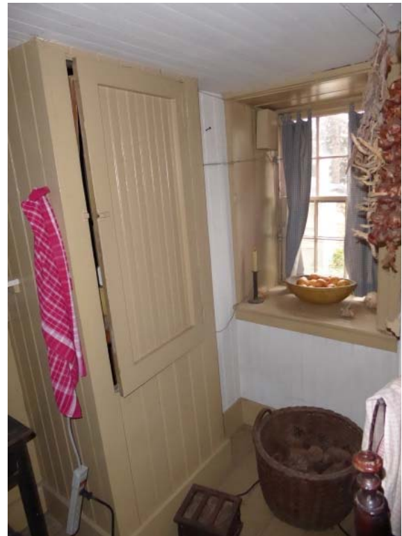
Photo 15: Dumbwaiter cupboard and window at northeast corner.
