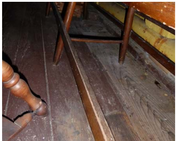
Photo 19: Flooring near north wall. Boards appear to have been replaced and are sagging down.
