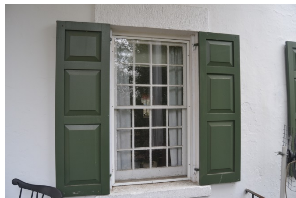
Photo 6: Typical first floor window at the main section of the house.
