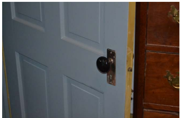
Photo 90: Close-up of door from bathroom to Room 205.
