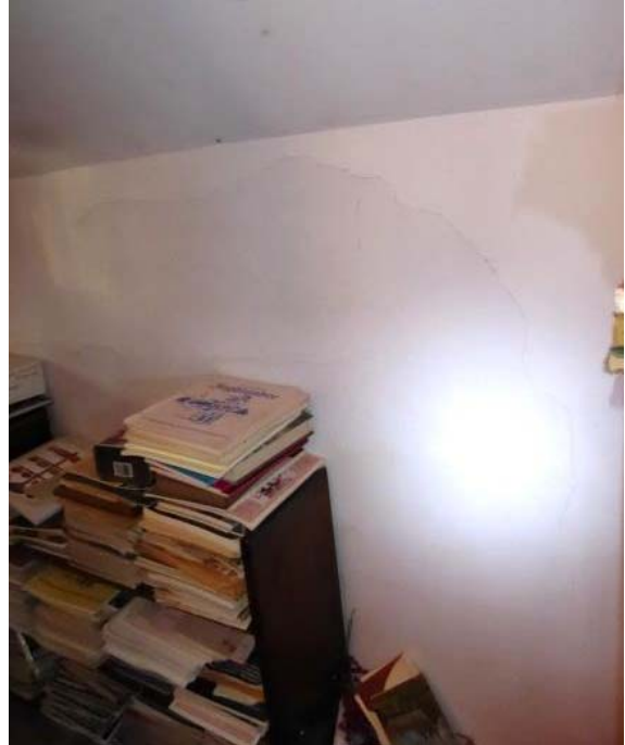
Photo 93: Looking towards north wall; cracks at wall and epoxy repair in sloped ceiling visible.
