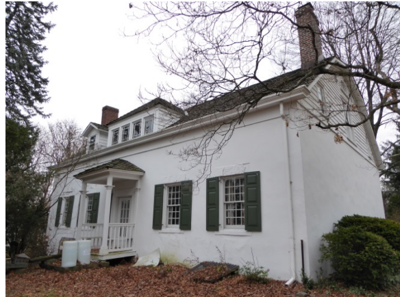
Photo 15: General view of the north elevation.
