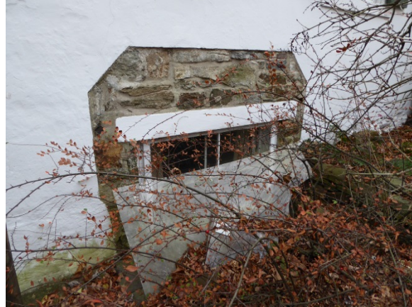
Photo 20: Left basement window. It is unclear why there is no stucco on the wall surrounding the window. Biological growth on base of wall at left.
