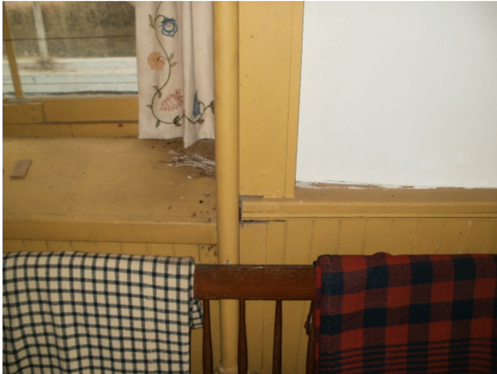
North basement wall finishes displaced from water infiltration and wall debris
