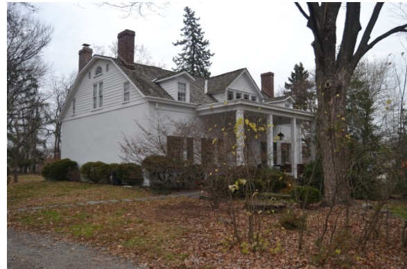
Photo 1: Overall view of the south façade from the southwest.
