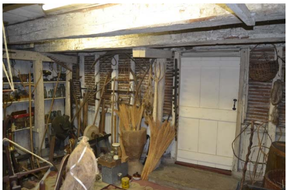
Photo 7: View north east. The door shown here is the door to Room 003. Note the post and bolster just to the left of the door.
