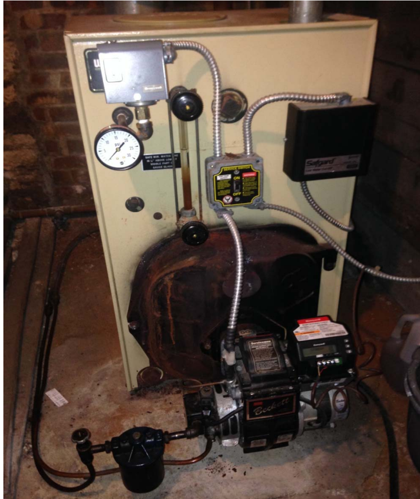
OIL FIRED STEAM BOILER
