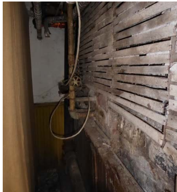
Photo 21: Mechanical space at northwest corner. Flooring is rotted and plaster is gone. Wood wainscot is painted a different color from the rest of the room.
