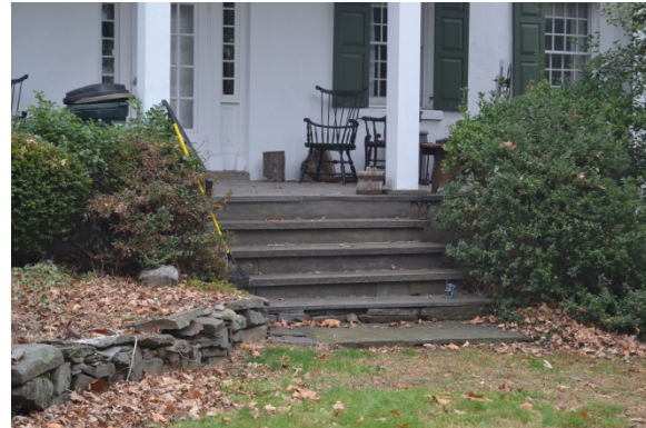
Photo 4: Front steps leading up to the porch from the south.
