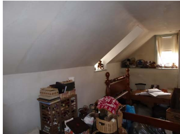
Photo 101: View of south and west walls. Dormer window at center.
