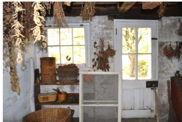
Photo 30: View south showing the door and window on this side. The door is in poor condition.
