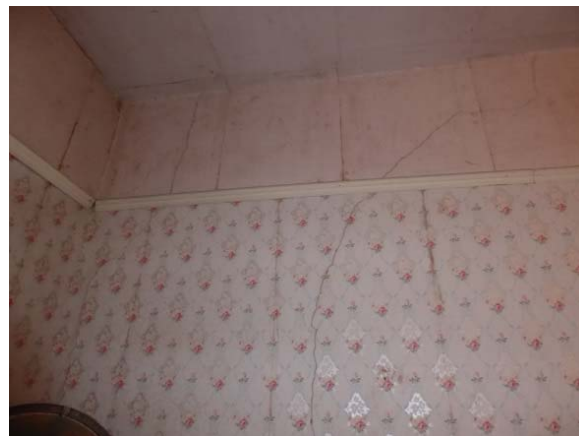
Photo 98: Cracks in wall at northwest corner.
