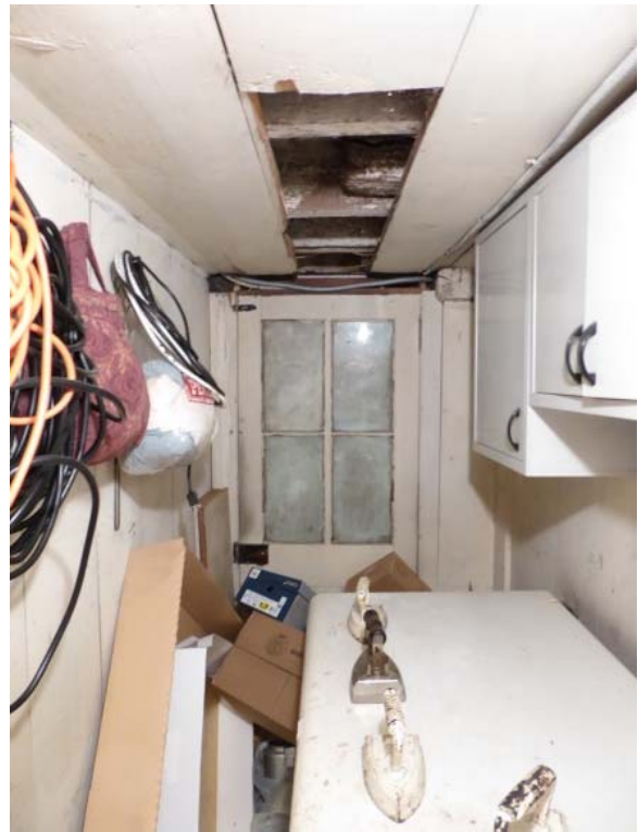
Photo 1: Looking east towards door to Museum Bedroom. A missing board in the ceiling reveals the continuation of the large timber joists above this space.
