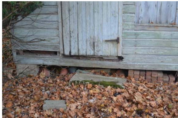
Photo 34: Close-up of the bottom of the east board-and-batten door.
