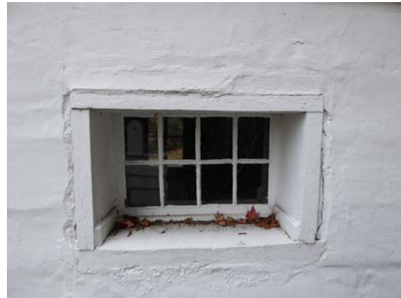
Photo 27: Eight-lite fixed window at north elevation of "smokehouse."
