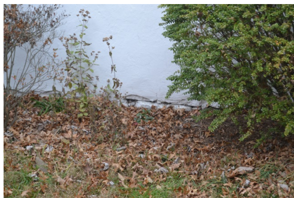
Photo 14: Area of exposed stone foundation at the base of the stucco on the west elevation.
