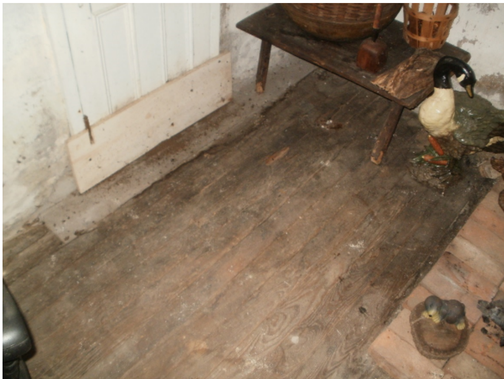
Water damage and buckled floor boards in smokehouse
