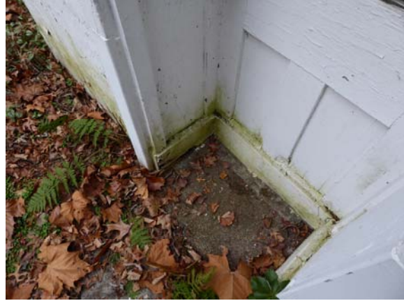
Photo 26: Door into "smokehouse." Note considerable water damage at the door and trim..
