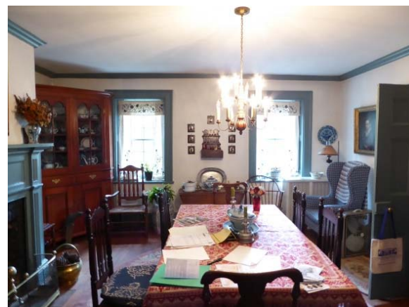
Photo 42: View of south wall in Room 102 showing windows.
