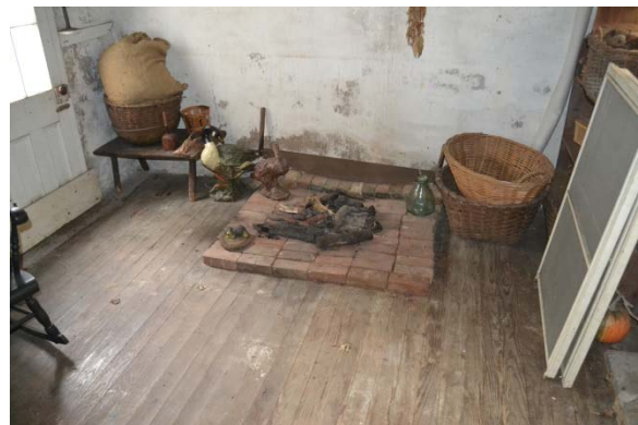
Photo 33: View of the floor showing a brick hearth, which along with the open fire remnants appear to be a later staging. At the right and left (south and north) the floor is very soft.
