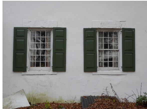
Photo 17: Stone lintels at right two windows are scaling. Bulge and cracking in stucco visible below both windows.
