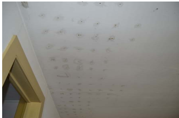
Photo 69: View of the ceiling showing unfinished epoxy ports for attachment of plaster to lath. This was done by the current owner.
