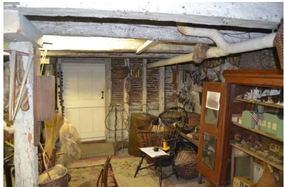
Photo 6: View east. The back side of the plaster walls and the door to Room 003 three are visible.
