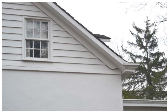
Photo 12: View of the south gambrel end roof slope and window.
