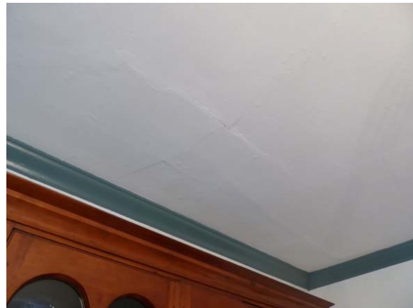
Photo 44: Cracks in plaster ceiling near northwest corner.
