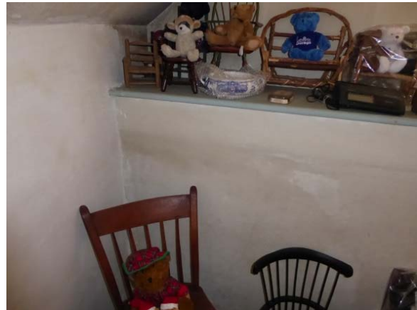
Photo 103: Plaster under ledge is uneven.
