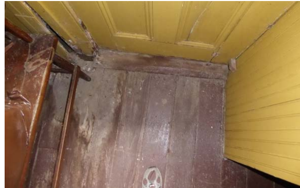
Photo 20: Staining and rotted wood at floorboards and exterior door frame. Cracked wood door panel.
