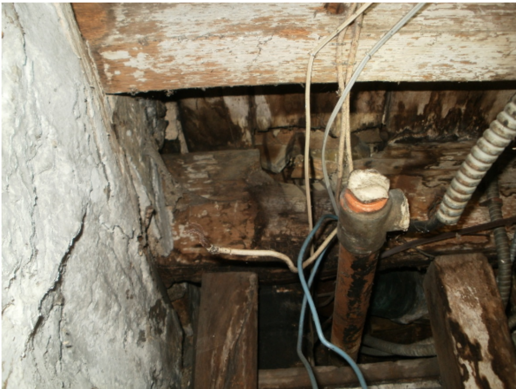
Water staining on first floor framing along north wall below second floor bathroom leak
