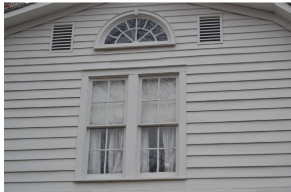
Photo 11: View of the arched fanlight at the attic and the paired four-over-four windows at the second floor.
