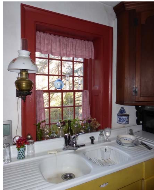
Photo 50: Twelve-over-twelve window at north wall and metal sink unit.
