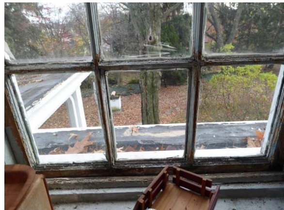
Photo 105: Detail of west window. Water damage to wood is visible.
