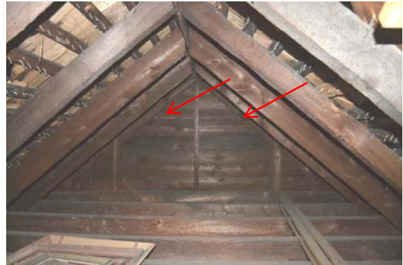
Photo 70: A system of pulleys in the attic provide a method of raising and lowering the two center sash at the large front dormer. There is no evidence that this system was operated from the second floor.
