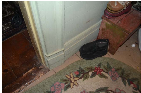
Photo 55: View of the baseboard with cap removed and replaced by a small quarter-round.
