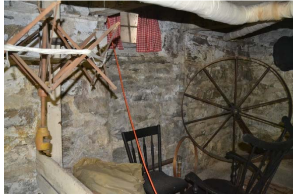
Photo 8: View into the southwest corner showing the vertical joints in the masonry where a door opening had been.
