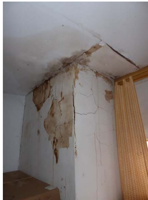
Photo 92: Plaster is failing at ceiling and walls of chimney bump-out.
